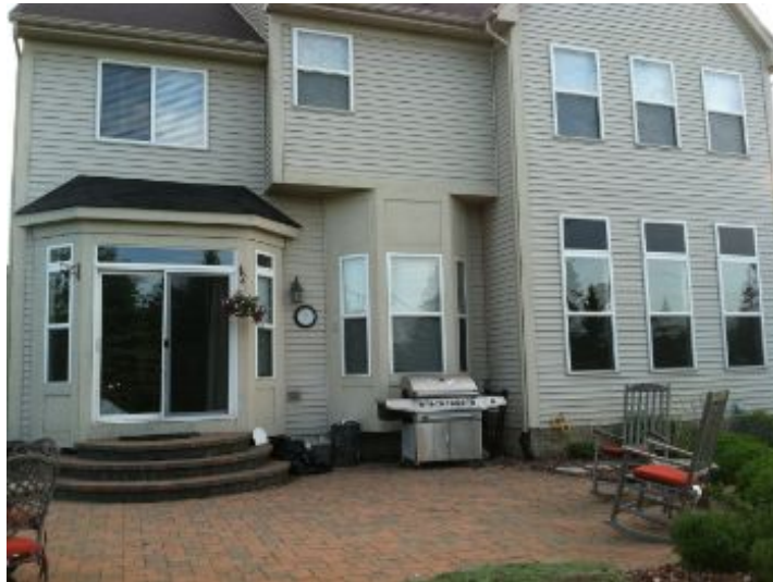
There were no railings installed at the steps. Location: back door
